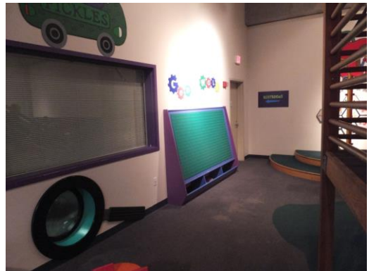
Figure 24 - Curved Wooden Platforms Block Access to Exit Doors in Polymer Funhouse Area
