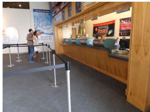
Figure 16 - Box Office Counter not Cane Detectable
