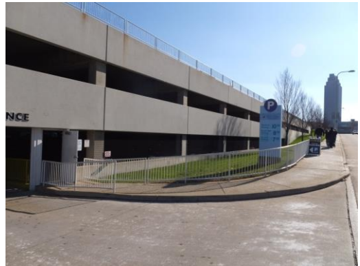
Figure 4 - Steep Approach and Limited Door Clearances
