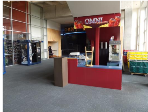
Figure 13 - Omnimax Concessions Counter Not Lowered at Cash Register
