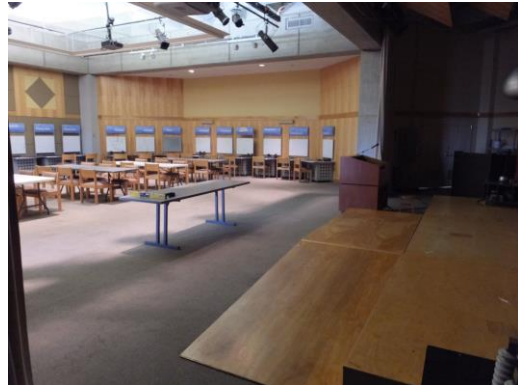
Figure 8 - Inaccessible Ramp at Reinberger Auditorium Stage
