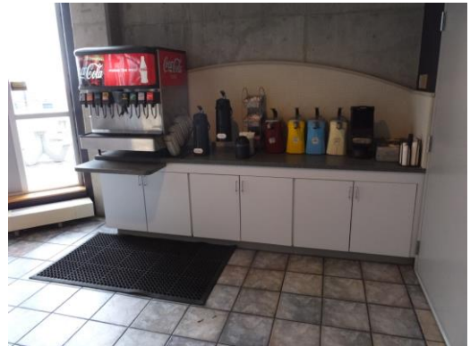
Figure 11 - Shelf Below Soda Dispenser is not Cane Detectable
