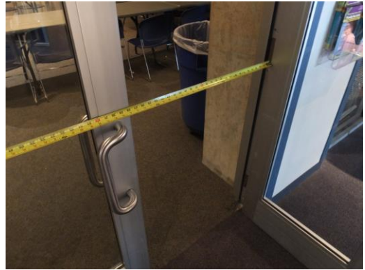
Figure 23 - Narrow Doors to Demonstration Lab B
