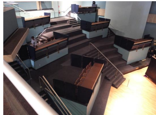
Figure 9 - Poor Sight Lines in Great Lakes Situation Room Auditorium
