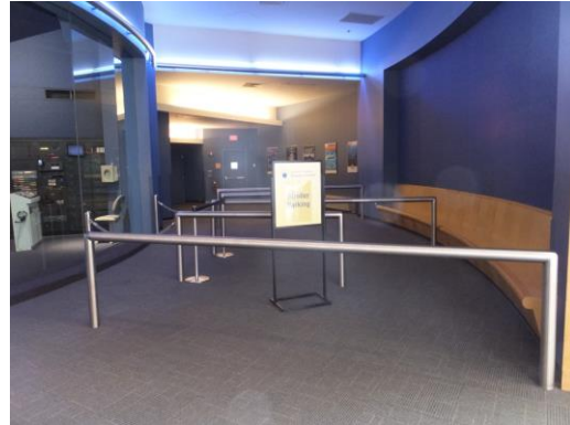
Figure 15 - Leaning Rails and Stanchions are not Cane Detectable
