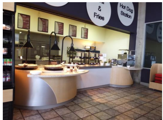
Figure 12 - Lowered Counters Not Cane Detectable
