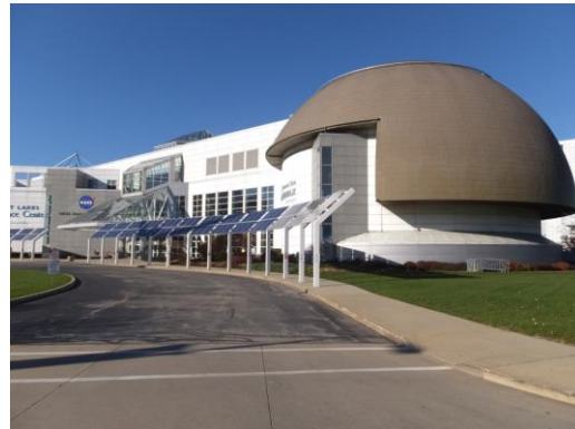
Figure 3 - Excessive Cross Slope along Route from Erieside Avenue
