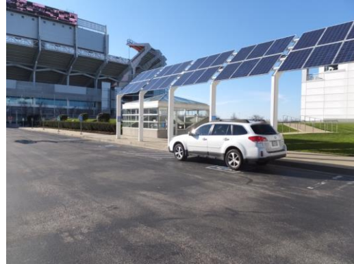
Figure 1 - Designated Accessible Parking in Drop-Off Driveway
