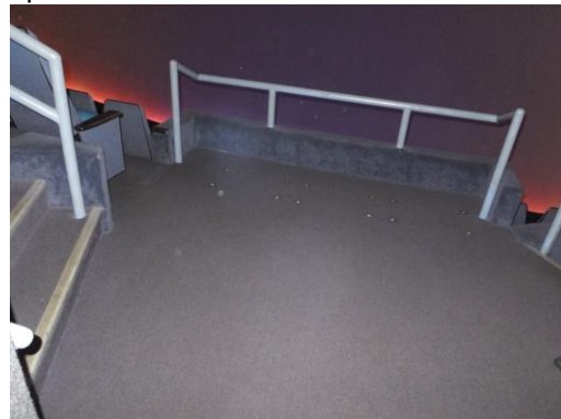
Figure 14 - Wheelchair Seating (Right Side) Area of Omnimax IMAX Theater has Posts and Stairs Encroaching
